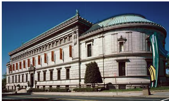
LEO A DALY recently completed phase one of George Washington University's Corcoran School of the Arts & Design, transforming the 1897 Ernest Flagg-designed gallery into a state-of-the-art home for arts education.
