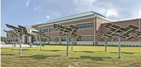
Solar panels promoting sustainability at Dickinson (Texas) ISD, Educational Support Center. Photo by Jud Haggard, courtesy of PBK.
